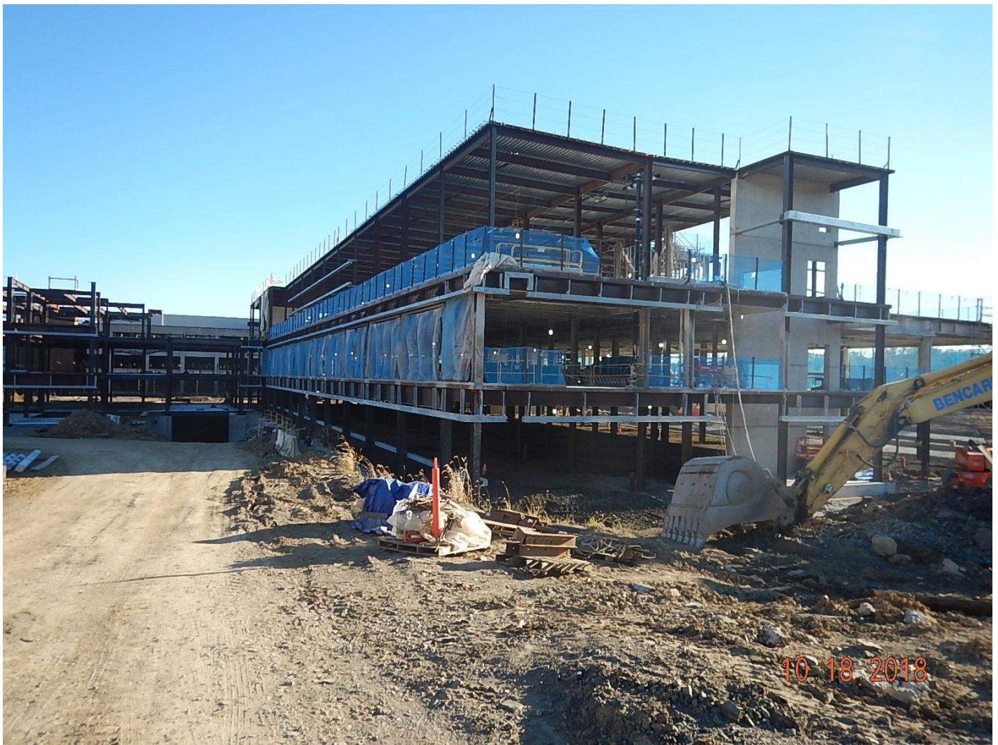
OVERALL CONSTRUCTION VIEW OF N BUILDING WITH PRECAST SHEAR WALL AND M BUILDING IN THE DISTANCE ON THE LEFT
